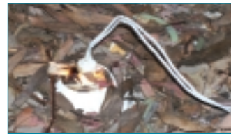
Leaves and debris brought in to ceiling space by birds or wind create fire hazard. Picture below shows fire protective cover installed over light
