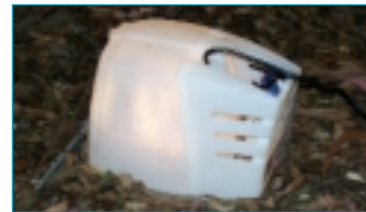
Leaves and debris brought in to ceiling space by birds or wind create fire hazard. Picture below shows fire protective cover installed over light
